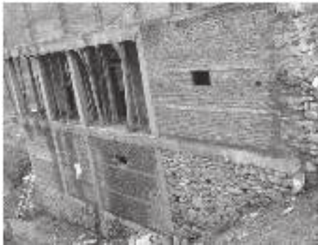
Fig. 14. RCC building with 230mm x 230mm column.
