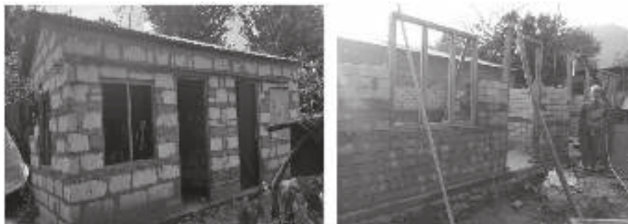
Fig. 11. Block masonry buildings in cement mortar (a) hollow concrete blocks (b) interlocking blocks.
