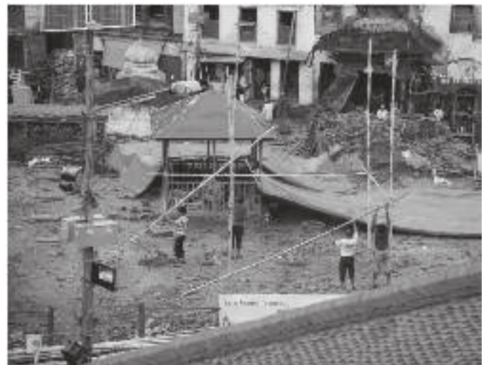
Fig. 13. Bamboo scaffold being assembled to cover the foundation of Kasthamandap from monsoon rain (Source: Rebuild Kasthamandap).
