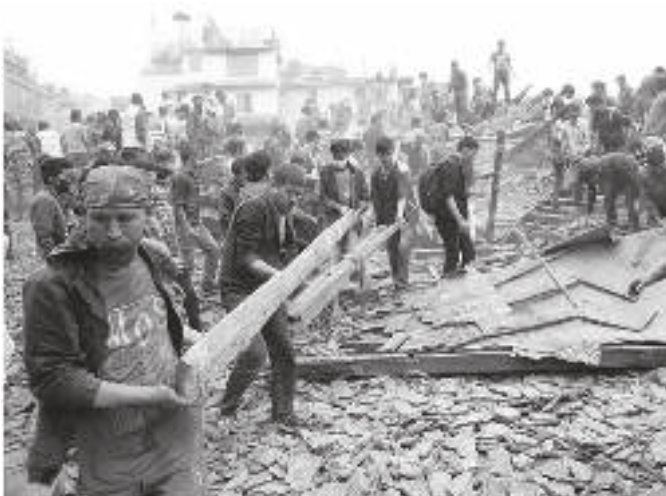
Fig. 9. Rescue work at Kasthamandap right after the earthquake (Source: http://ecs.com.np/features/why-kasthamandap-matters ).
