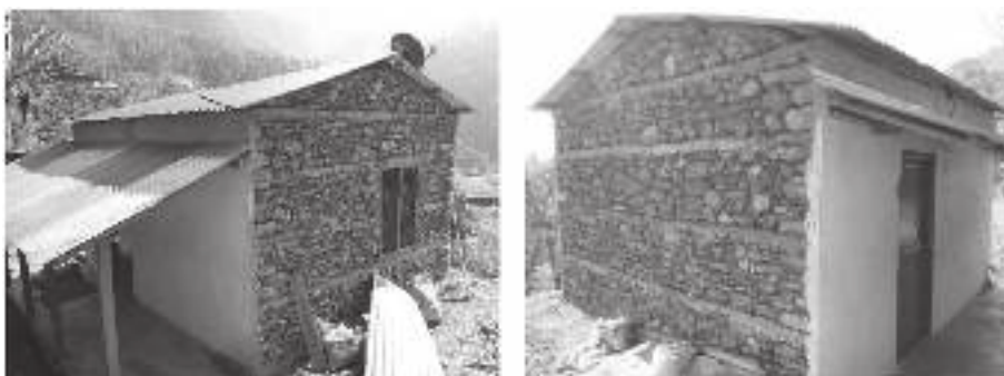
Fig. 6. One room building with stone in mud mortar and flexible roofing.
