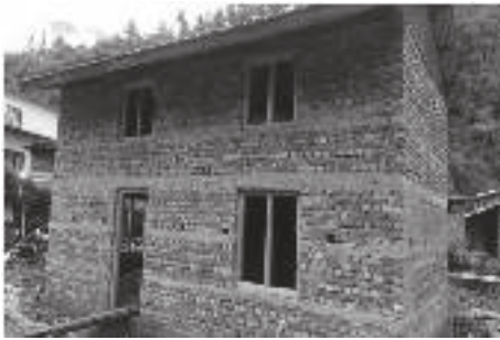
Fig. 19. Brick masonry building.
