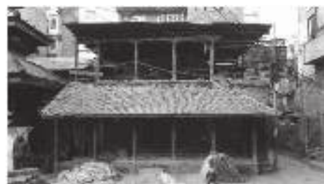
Fig. 13. Om Bahal Seto Ganesh Guthi ghar after 2015 earthquake.
