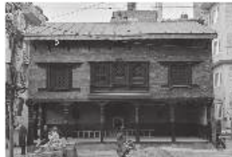
Fig. 11. Construction completion of new Bhagavati Phalcha, Date: Feb 2021.
