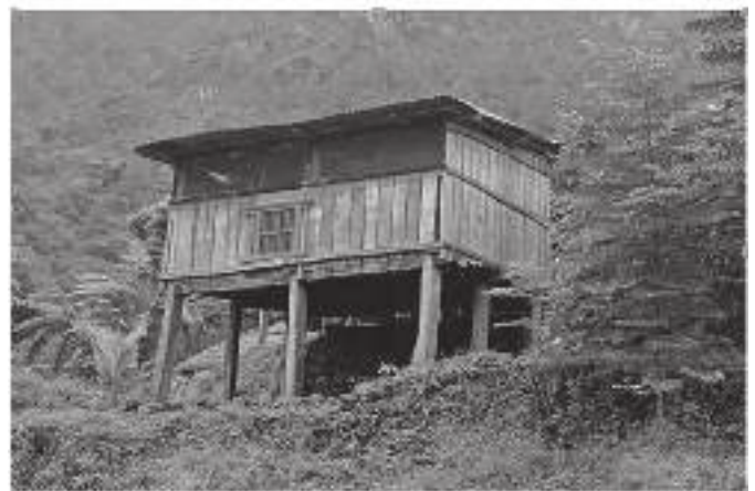
Fig. 3. Goat shelters with different materials constructed by beneficiaries using cash transfers and adopting improved designs. Photo by CRS staff.
