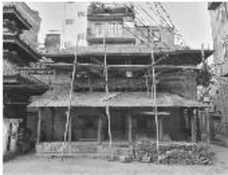
Fig. 15. On-going construction of Om Bahal Seto Ganesh Guthi ghar, Year:- Feb 2021.
