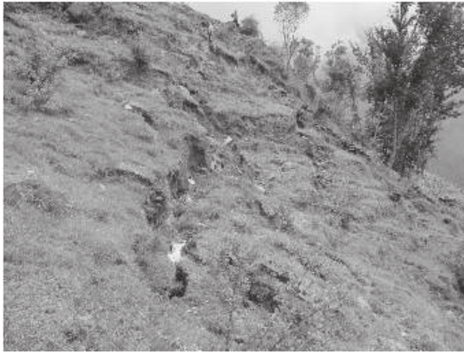
Fig. 6. Open cracks observed in the ground situated up slope from the Kalche settlement (Silwal [26]).
