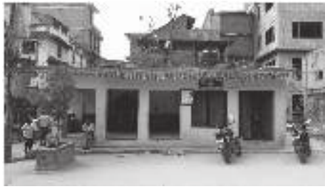
Fig. 7. Bhagavati Phalcha – Kobahal with modern RCC building, Year:- 2017.
