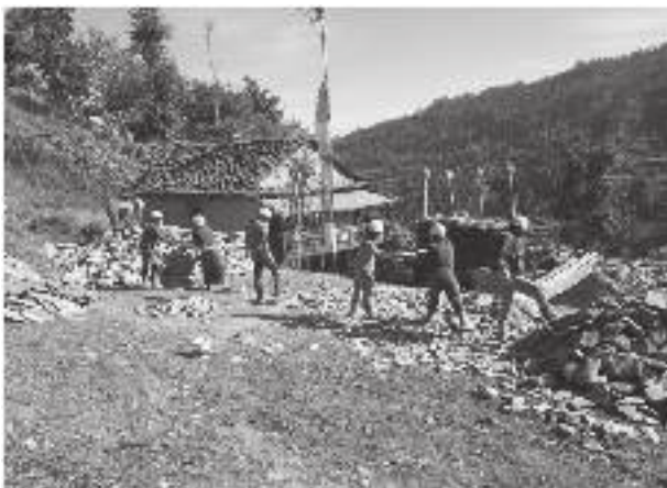
Fig. 10. Cluster members involved in demolition activities and classifying the salvaged materials.
