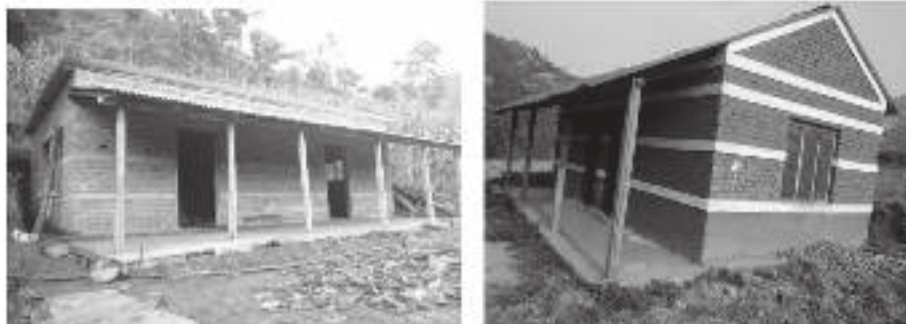
Fig. 8. Single story brick masonry building in cement mortar.
