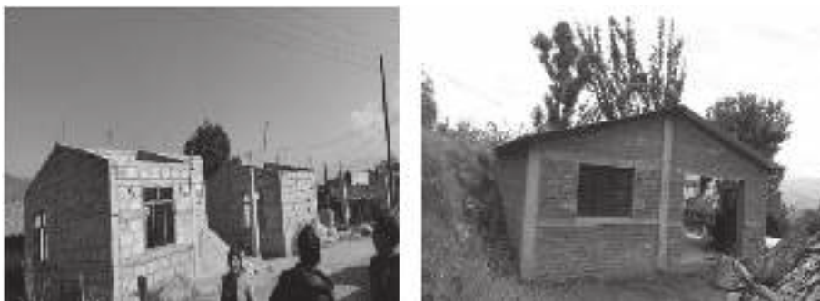
Fig. 4. Column building structures with (a) concrete blocks in cement mortar (b) bricks in cement mortar.
