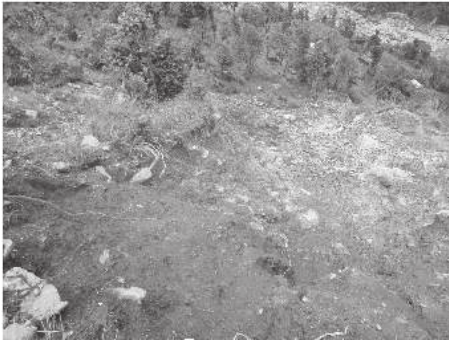
Fig. 8. Landslide on the upslope of Chihan Dada (Silwal [26]).
