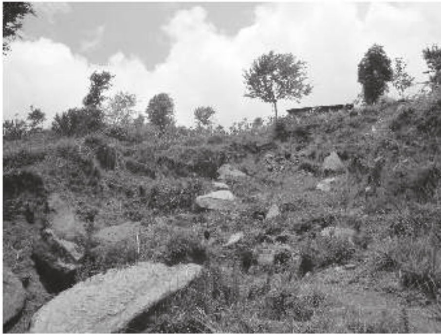
Fig. 10. Failed terraces and boulders on down slope of house [41].
