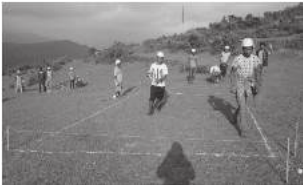
Fig. 13. Mason Training to community members-Practical exercise on layout of building.
