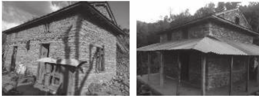
Fig. 7. Two-story stone masonry building in mud mortar.
