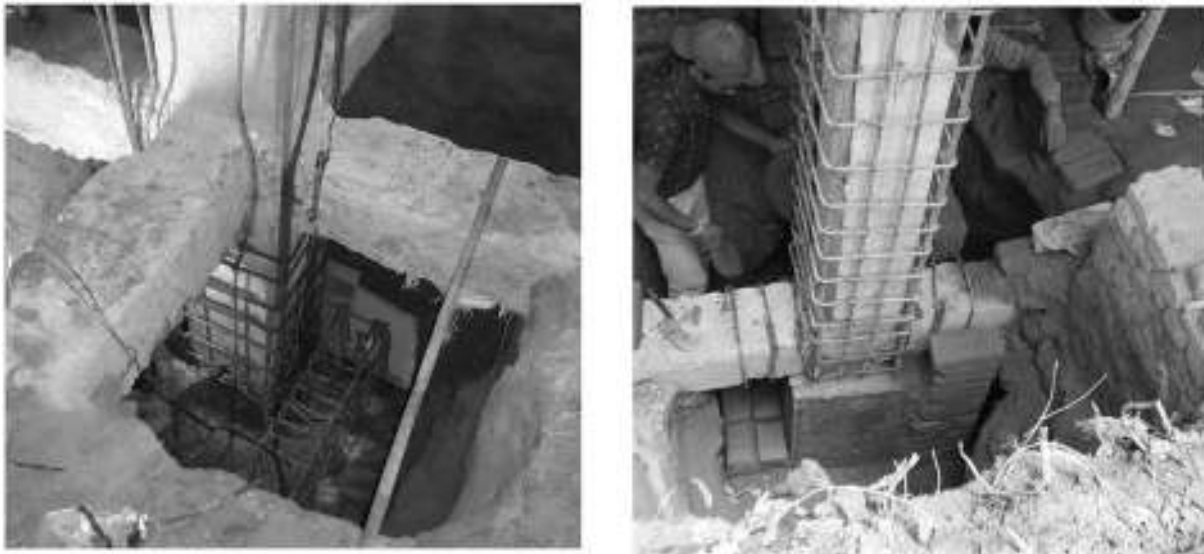
Fig. 20. Installation of base for column jacking.
