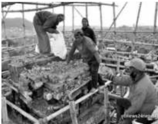
Fig. 34. Dismantling of top floor.
