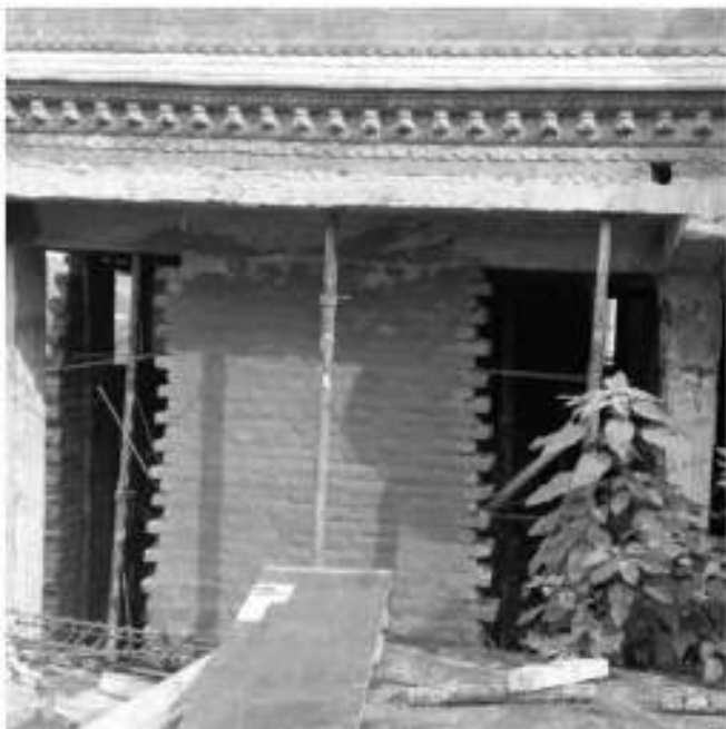
Fig. 11. Brick wall under the beams.
