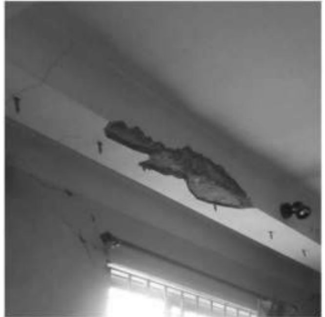
Fig. 9. Nozzles for epoxy grouting at beam.
