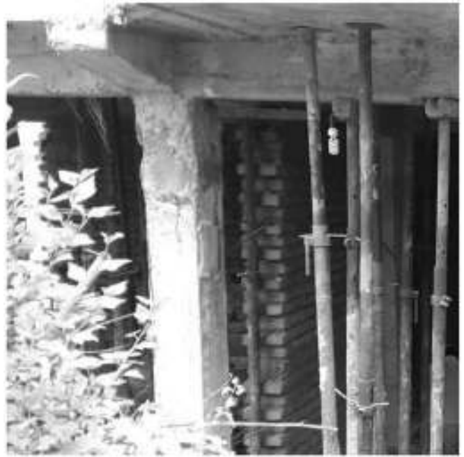
Fig. 8. Epoxy grouting and support at column 2A.
