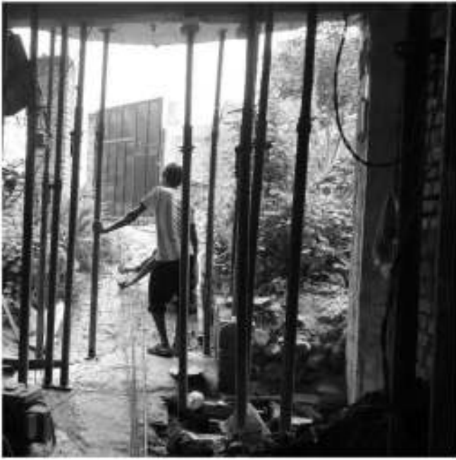
Fig. 10. Metallic props under the first-floor slab.
