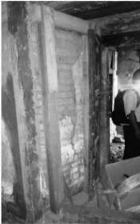
Fig. 33. Strengthening of walls in first floor.
