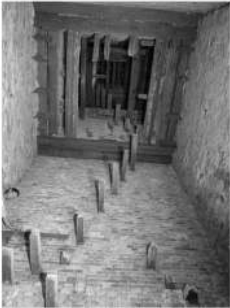
Fig. 5. Open floor system in Nyatapola temple.
