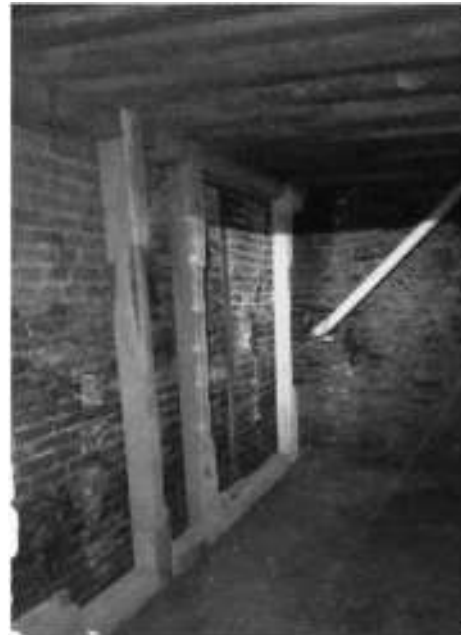
Fig. 32. Strengthening of structure in ground floor.
