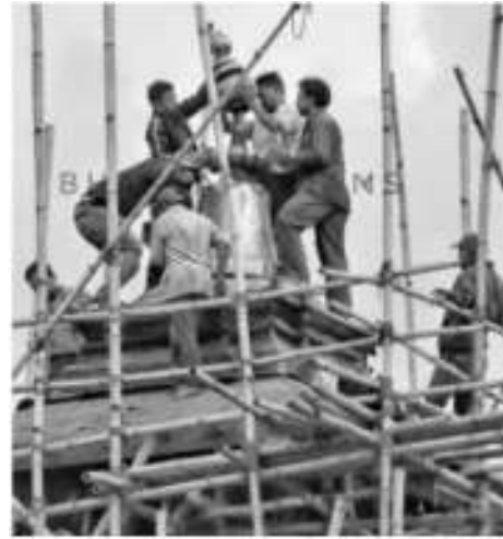
Fig. 36. Placing pinnacles on top roof.
