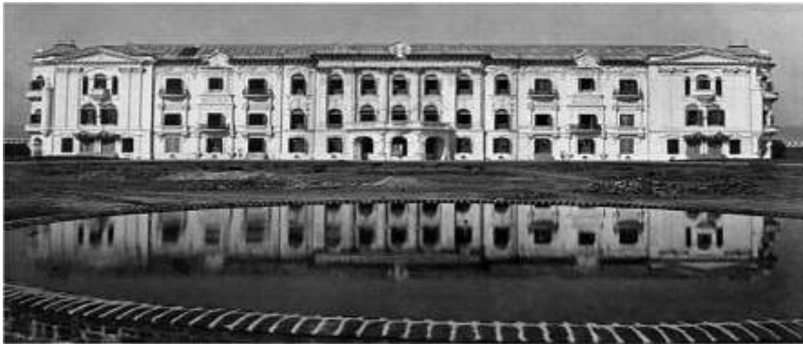
Fig. 3. East elevation of Shital Niwas before 1934 CE Earthquake (Source: Nepal Archives, DOA).
