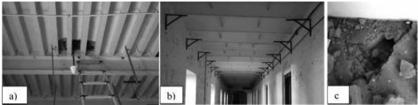
Fig. 5. a) Timber floor above steel I-section girder b) Jack-arch floor supported in steel I-section beams above corridor c) Brick and mud layer in the floor above joists.
