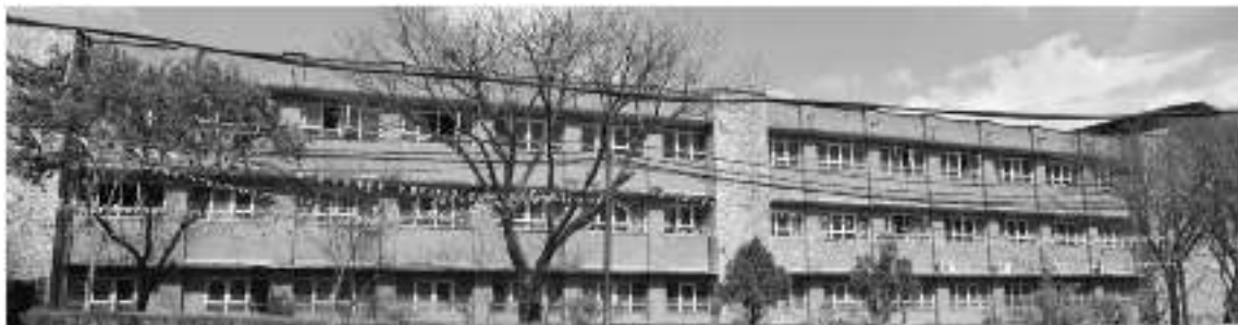
Fig. 2. D block- south elevation of the Department of Mechanical Engineering.
