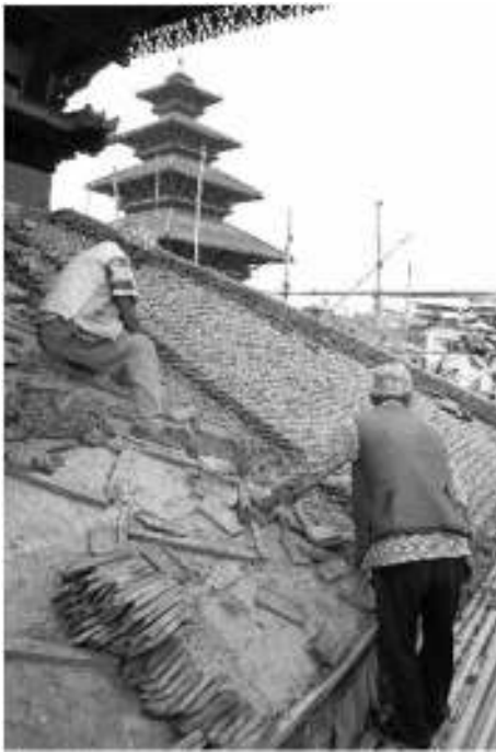
Fig. 15. Laying out jhingati in the roof of Bhairavnath temple.
