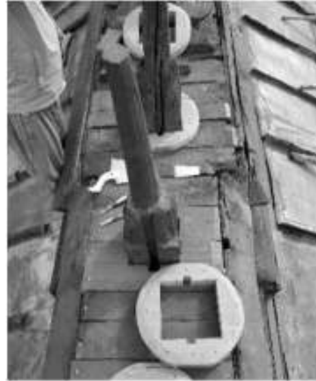
Fig. 31. Replacing the decayed wood by new ones.
