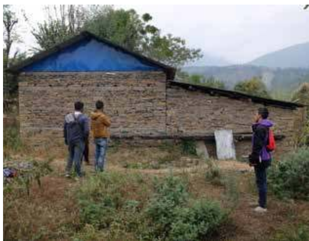
Figure 19.1: ASF-Nepal, SMM: Extension with earthquake resilient elements after receiving third tranche.
