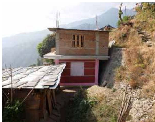
Figure 19.2: ASF-Nepal, RCC house: Extension after receiving a third tranche.
