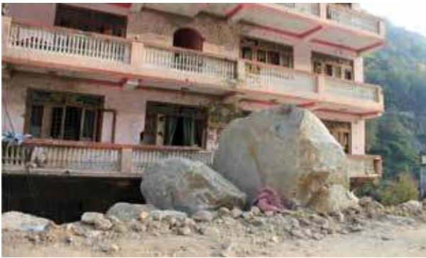
Figure 37: Many large boulders and debris flow splash on buildings of Liping. View to E
