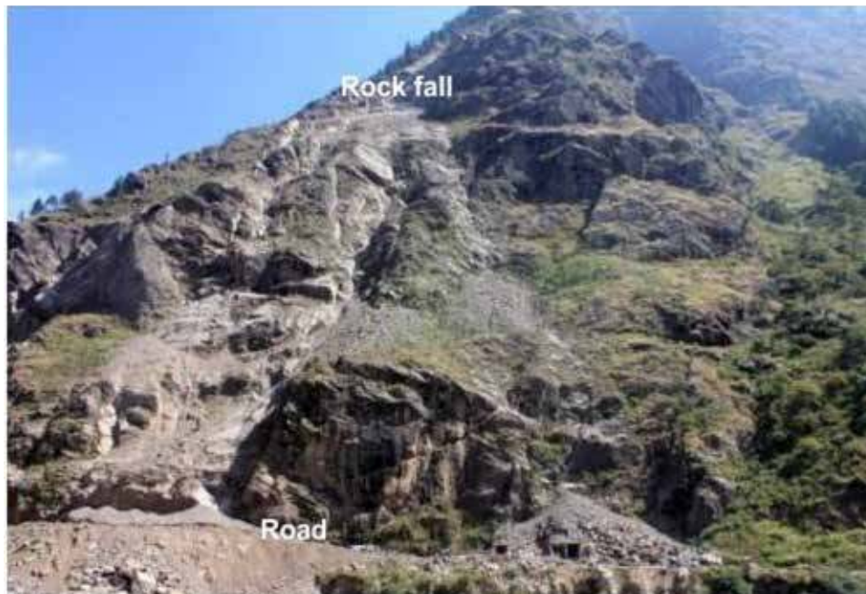
Figure 16: Massive rock fall near Friendship Bridge of Rasuwa Gadhi. View to NE
