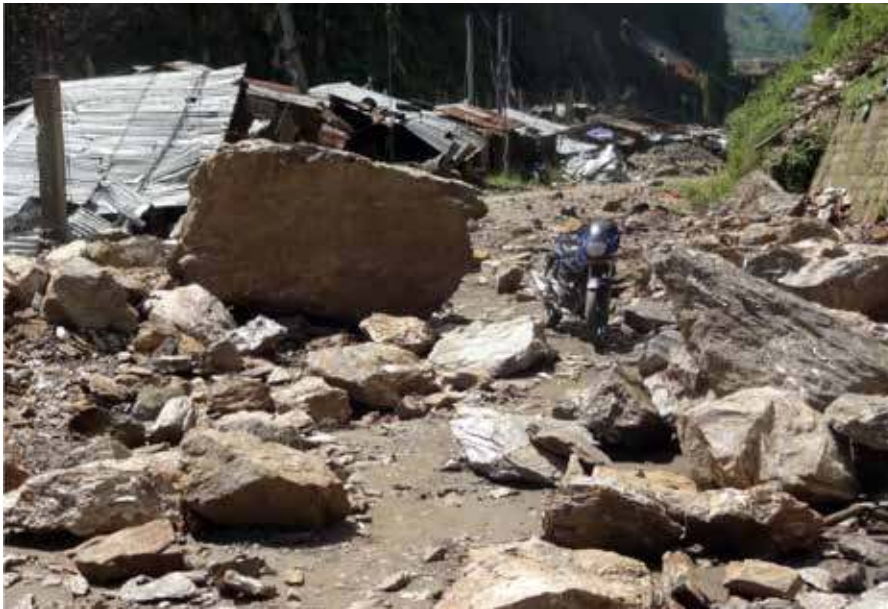
Figure 35: Failed rock blocks at Larcha, damaging settlement and road. View to S
