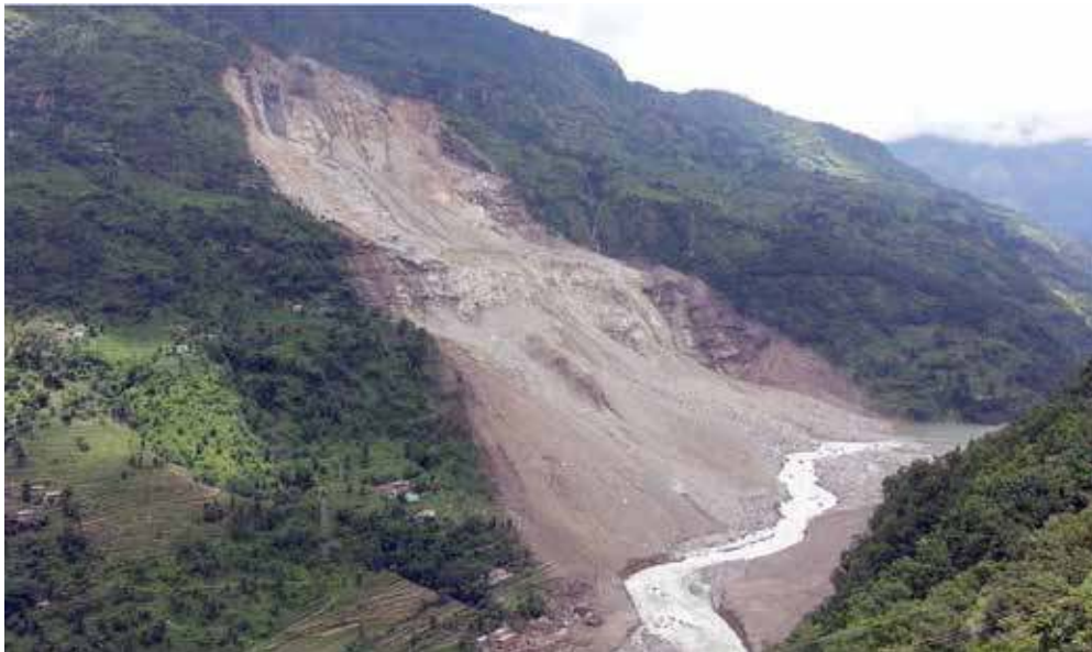
Figure 52: Jure rock avalanche on Arniko Highway. View to N
