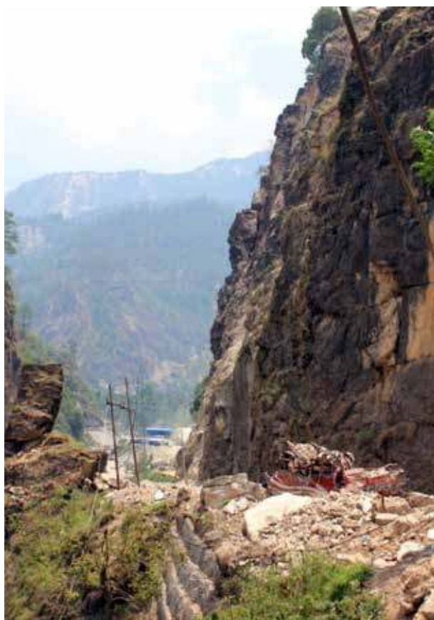
Figure 28: Unstable rock cliff with vertical joints near Chaku, where rock falls destroyed a vehicle. View to N
