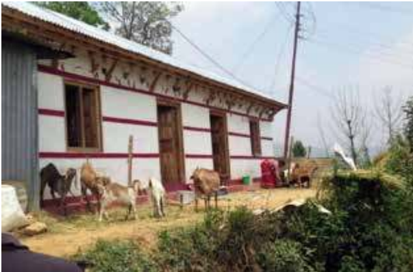
Picture 5: Model house constructed by Caritas Nepal for two widows. Location: Balthali, Panauti -11, Kavrepalanchowk. Photo: Caritas Nepal
