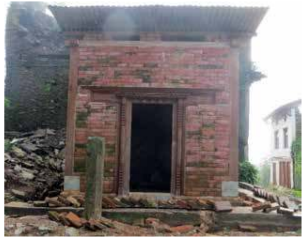
Picture 4: Narayan Temple after reconstruction
