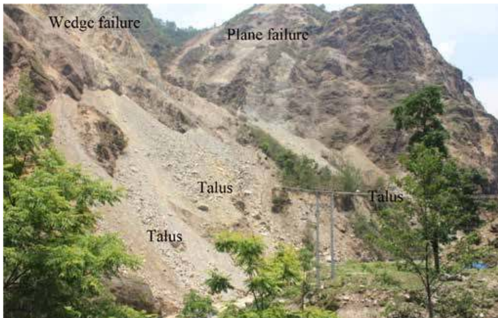
Figure 31: Shallow rockslides, rock falls, and talus cones opposite Chaku in Bhote Koshi River. View to NW
