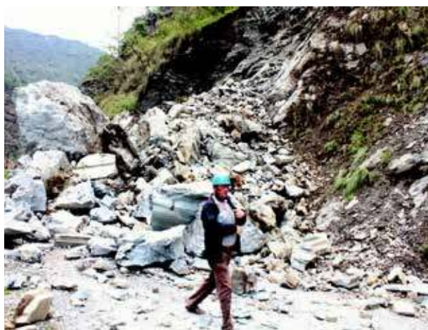
Figure 27: Wedge rockslide with large boulders, blocking Arniko Highway. It was triggered by first heavy monsoon rain after earthquake. View to NW
