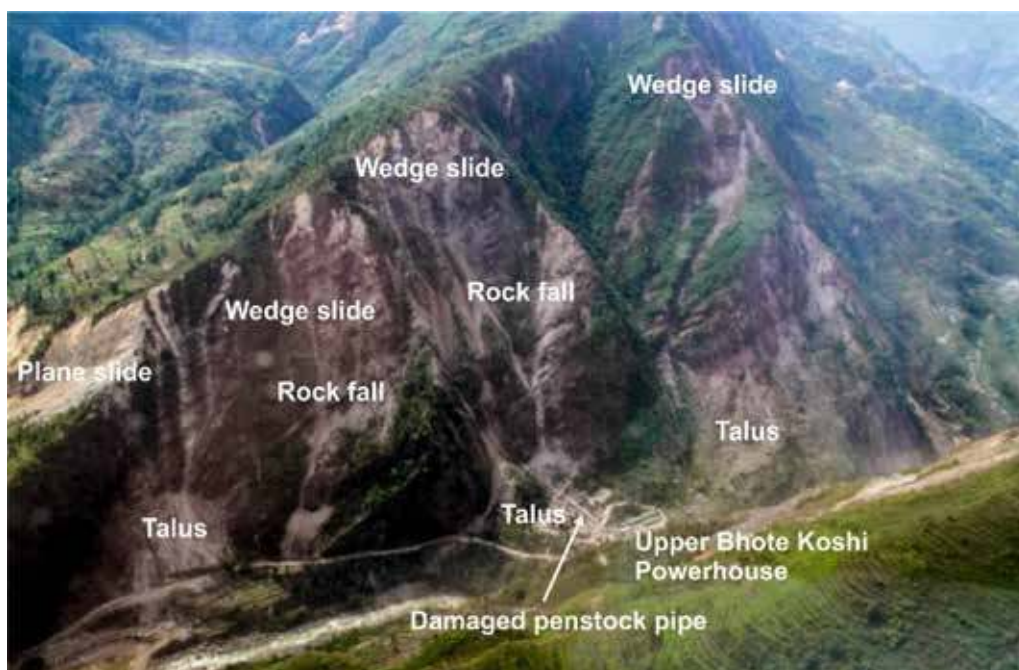
Figure 33: Coseismic mass movements developed on rock cliff adjacent to Upper Bhote Koshi Powerhouse. Three joint sets are prominent. Rock falls damaged powerhouse and penstock pipe. View to ESE
