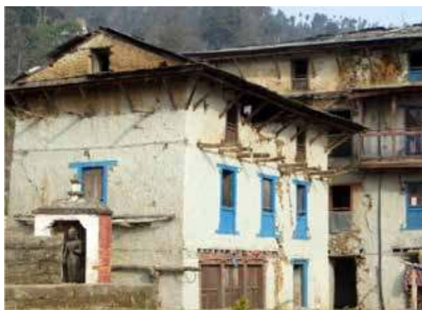
Picture 7: Houses damaged by 2015 earthquake
