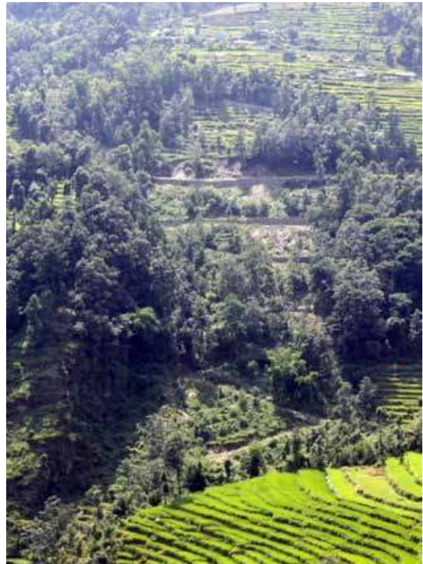
Figure 39: Soil slide at Km 10+500 of Upper Tama Koshi Road. View to W
