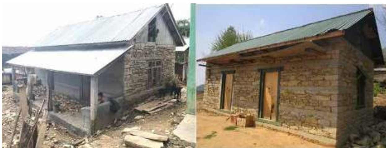
Figure 9: Left: demonstration house in Aru Pokhari, Gorkha supported by an INGO working in the area. Right: a house constructed as part of on-the-job training for masons in Kavrepalanchok supported by an INGO. Source: HRRP, 2020
