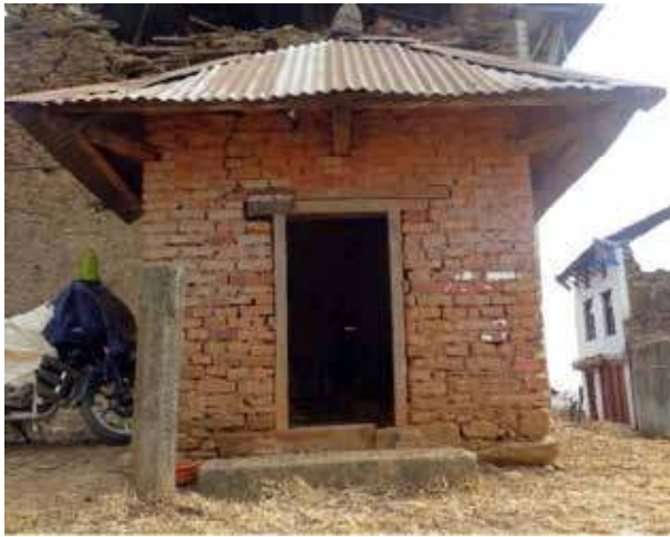
Picture 3: Narayan Temple after Gorkha Earthquake 2015
