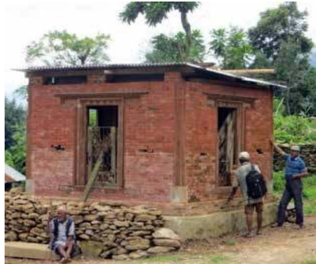
Picture 6: Re-constructed Pashupati Temple
