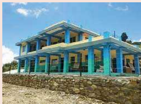
Photo 34: Reconstruction of health post at Lamachaur, Kaski
