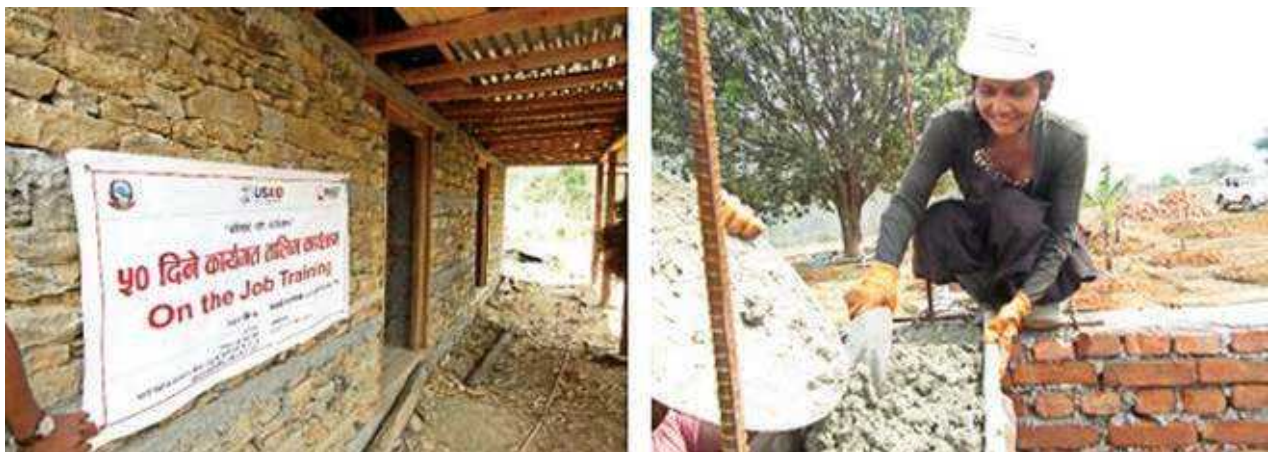
Photo 22: Female masons practicing concretizing during an on-the-job training
