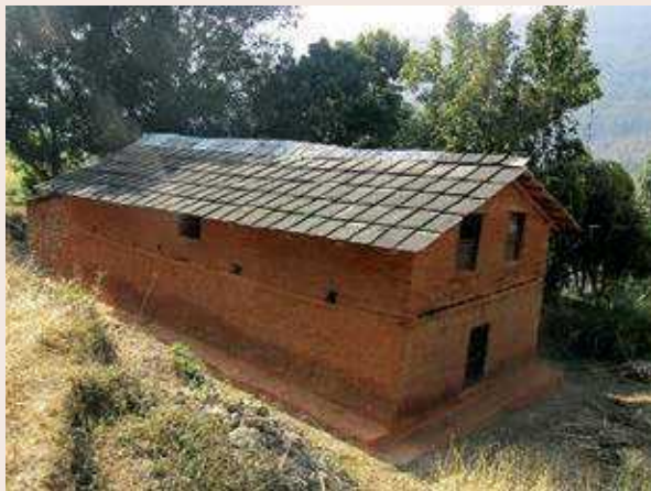
Photo 1: Stone masonry in mud mortar, slate/ shingle roofs
