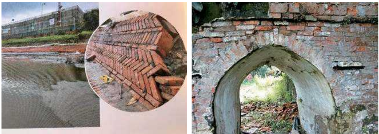
Embankment wall around pond
