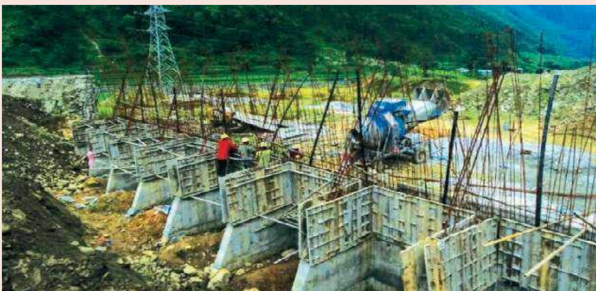
Photo 48: Trishuli 3A Hub (Under Construction)
