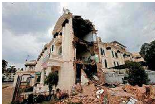
Collapse of south west corner
