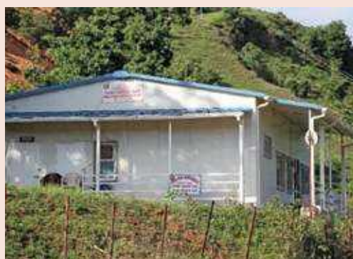
Photo 35: Reconstructed health post in Nalang, Dhading
