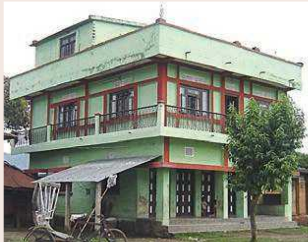
Photo 6: Reinforced concrete frame structure houses
