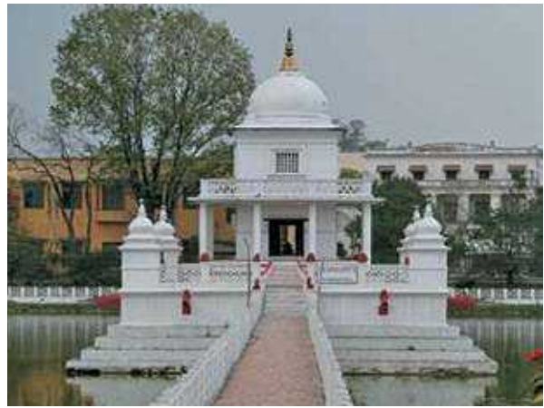
FIGURE 52: : RANIPOKHARI AND BALGOPALESHWAR TEMPLE BEFORE THE EARTHQUAKE
