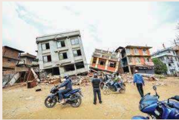
Photo 8: Debris management (Photo: Sandeep Gurung, 2015)
