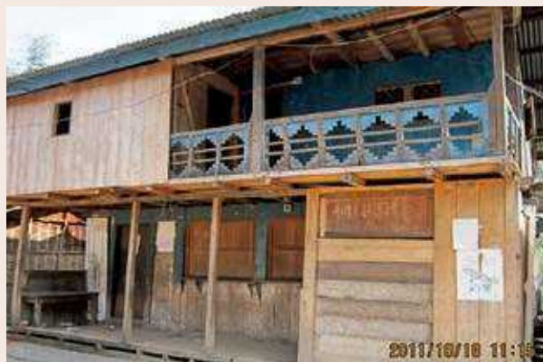
Photo 4: Timber frame houses
