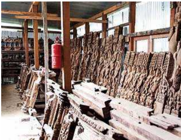
FIGURE 64: LEFT: THE SALVAGED WINDOW PARTS OF VARIOUS TEMPLES AND CARVED TIMBER ELEMENTS AND STRUTS WERE STORED IN A NEWLY BUILT SHED. PHOTOGRAPH: KVPT. JUNE 07, 2015. RIGHT: CARVED ELEMENTS WERE SORTED AND ASSEMBLED, AND ALL COMPLETE SETS FROM THE PILE OF RESCUED ELEMENTS WERE PLACED IN STORAGE. PHOTO: KVPT. MAY 02, 2015.
