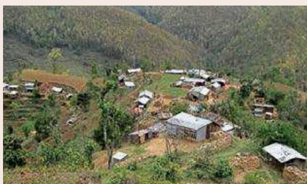
Photo 17: Damaged area with transitional shelters (2016) (Source: NSET)
