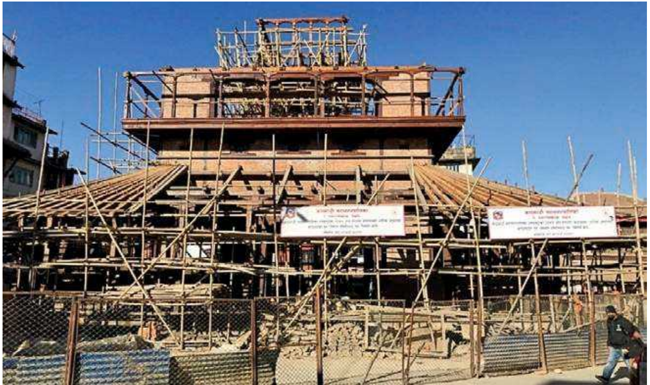
FIGURE 78: RECONSTRUCTION OF KASTHAMANDAP, PHOTO TAKEN ON 25 DECEMBER 2020
