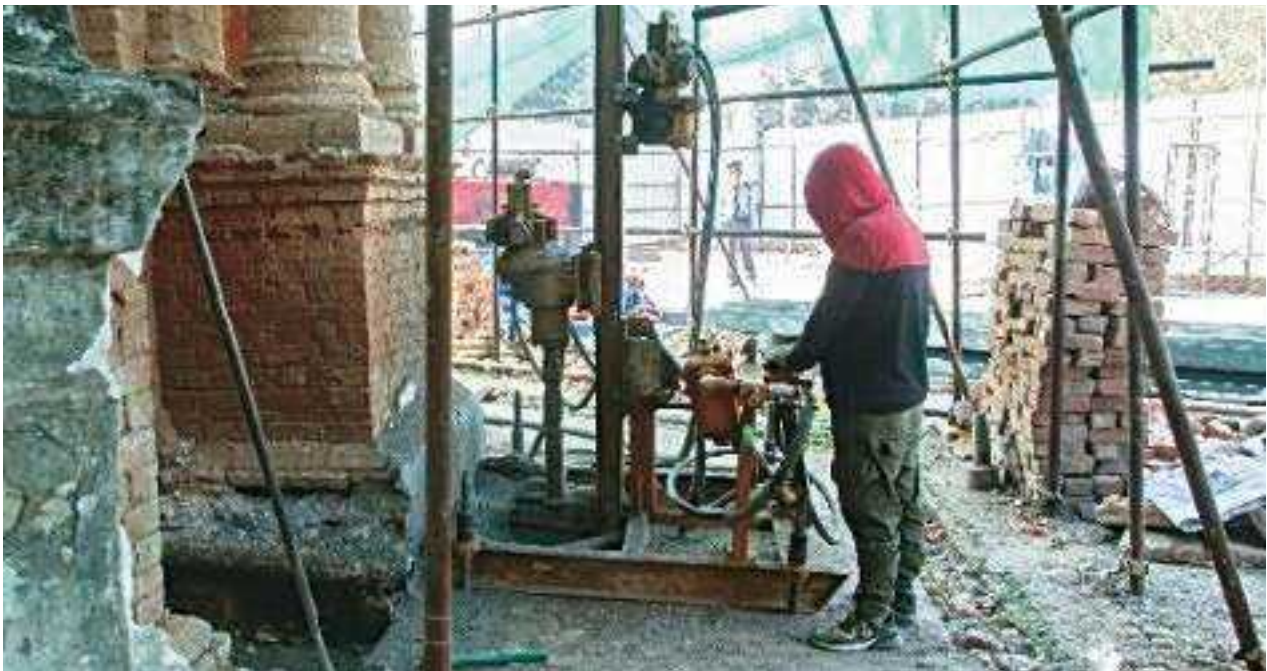
FIGURE 38: EXCAVATION FOR MICRO PILLING
