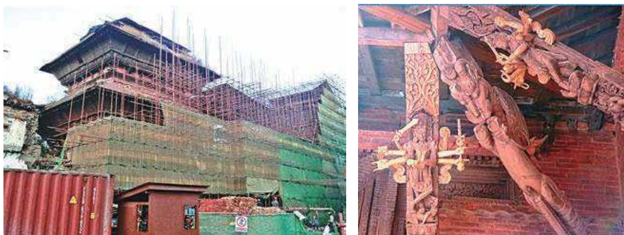
FIGURE 58: RECONSTRUCTION WORK AT THE TOWER COMPLEX (LEFT: SCAFFOLDING FOR RECONSTRUCTION AND RIGHT: INTRICATE DETAILING IN STRUTS PRESERVED)
