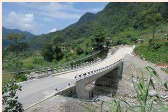
Photo 46: Reconstruction of bridges
