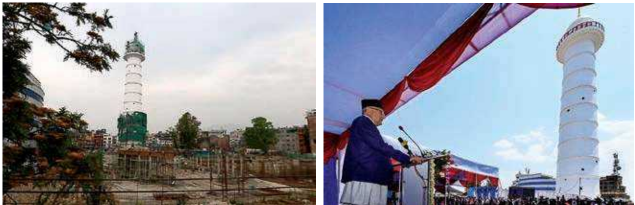
FIGURE 75: RECONSTRUCTION OF DHARAHARA TOWER WHICH WAS INAUGURATED BY THE RIGHT HONOURABLE PRIME MINISTER. (NRA,2021)
