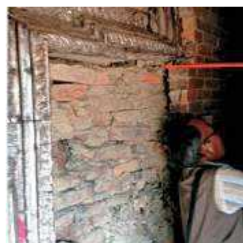
Separation inner and outer wall
