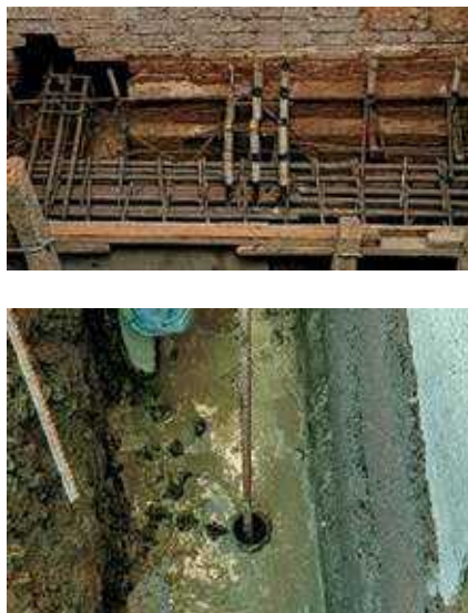
FIGURE 39: INSERTION OF METAL ROD INSIDE METAL PIPE & ANCHOR BOLT
