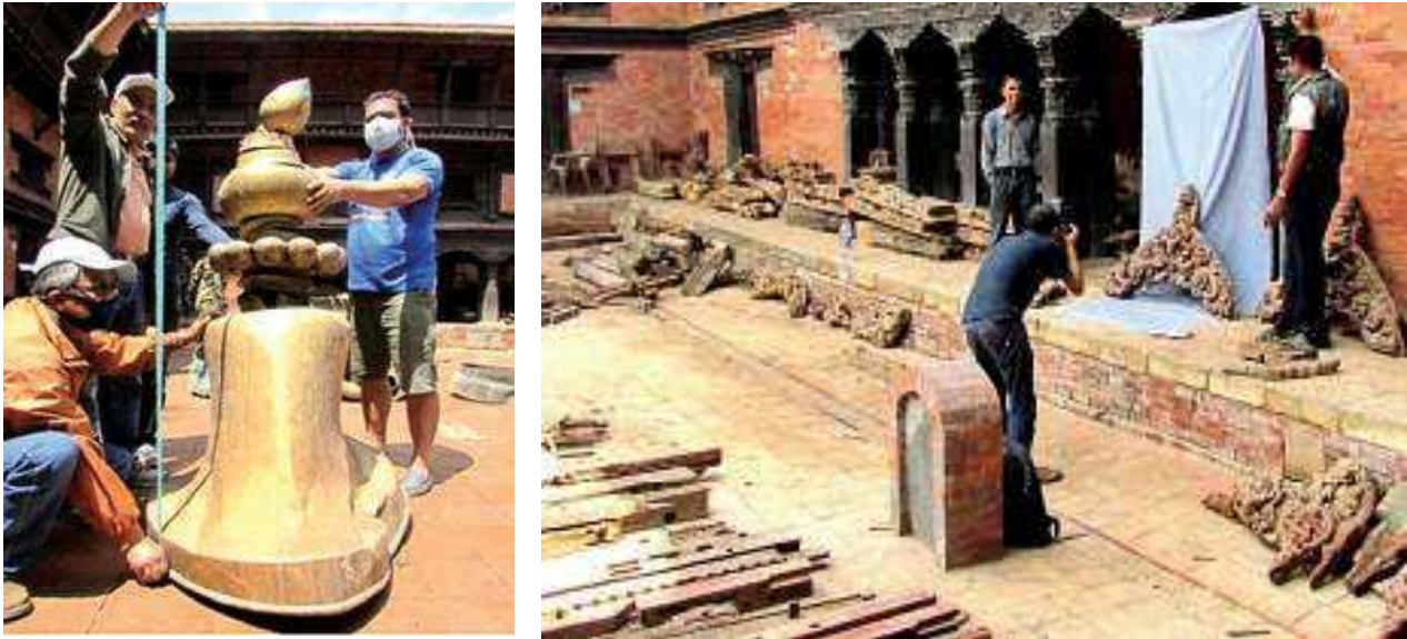
FIGURE 65: LEFT - DAMAGED PARTS WERE INDIVIDUALLY MEASURED AND PHOTOGRAPHED AS SOON AS THEY WERE TRANSFERRED TO A SAFER ZONE. PHOTOS: R. RANJITKAR, MAY 07, 2015 (RIGHT) AND MAY 09, 2015 (LEFT).
