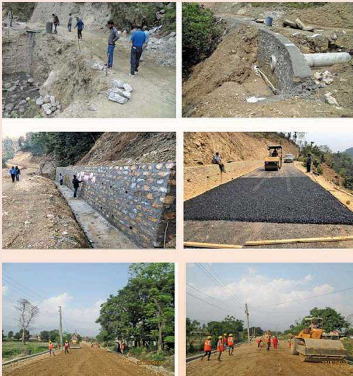
Photo 45: Civil and bio-engineering structures for slope protection (a. Lamjung Road; b. Kavre Road; c. Khurkhure Highway-Samitar-Thakuri Bhanjhyang Road)
