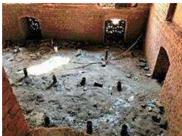
Ongoing micro pilling in an inner room of the building
