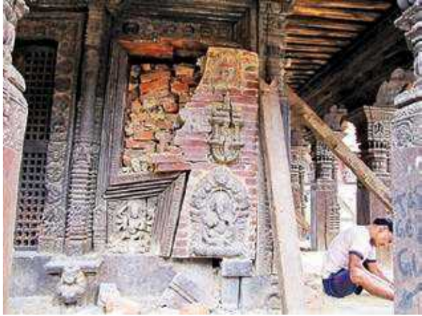
FIGURE 63: LEFT: VISVESHVARA TEMPLE, PATAN DURBAR SQUARE. TEMPORARY TIMBER SUPPORT WAS FIXED AT THE MONUMENTS THAT FACED STRUCTURAL RISKS. PHOTOGRAPH: R. RANJITKAR. MAY, 2015. RIGHT: NORTH TALEJU TEMPLE'S ROOF WAS DISLODGED. SCAFFOLDING WAS STARTED WITHIN A WEEK OF THE EARTHQUAKE AND THE TOP TIER WAS SECURED TO PREVENT FURTHER DAMAGE TO LOWER ROOFS. SOLDIERS ARE SEEN IN THE BOTTOM TRANSFERRING RESCUED BRICKS FROM THE SQUARE TO THE BACK GARDEN. PHOTO: R. RANJITKAR. MAY 10, 2015.
