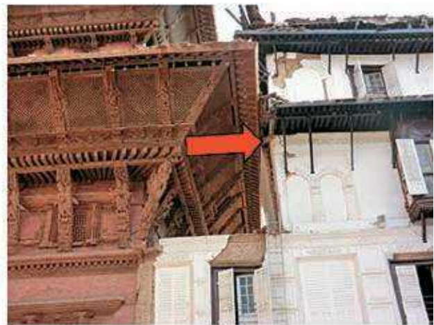
FIGURE 56: DAMAGES IN THE TOWER COMPLEX AFTER THE EARTHQUAKE
