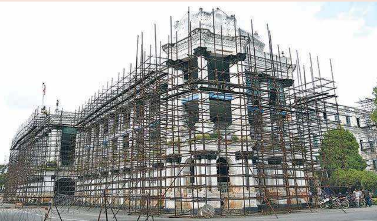
Photo 31: Retrofitting of Singhadurbar (South Lounge)
