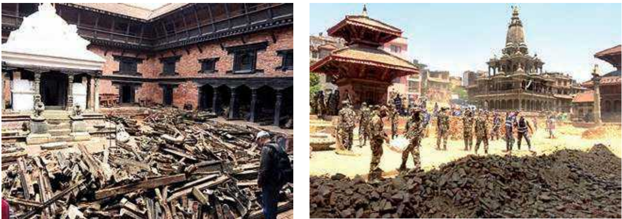
FIGURE 62: LEFT: ALL CARVED ELEMENTS FROM COLLAPSED MONUMENTS WERE CARRIED FROM THE DESTROYED SITE AND KEPT IN THE PATAN MUSEUM COURTYARDS. PHOTOGRAPH: R. RANJITKAR. APR. 30, 2015. RIGHT: UNUSABLE DEBRIS WAS COLLECTED FOR TRANSPORT TO A DUMPING SITE AFTER REUSABLE BRICKS WERE STACKED IN THE SQUARE. PHOTO: R. RANJITKAR. MAY 01, 2015.
