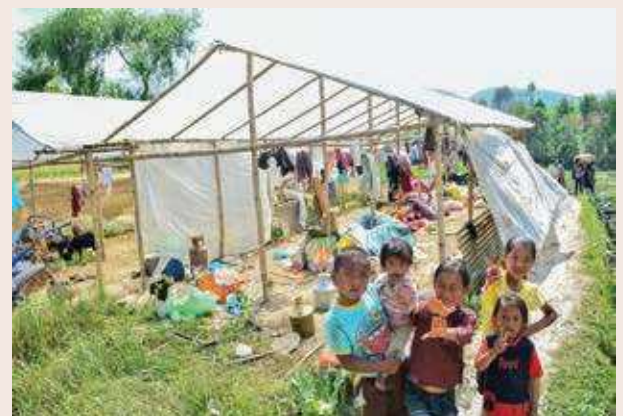
Photo 14: Temporary shelter with plastic sheets (Photo: Sandeep Gurung, 2015)
