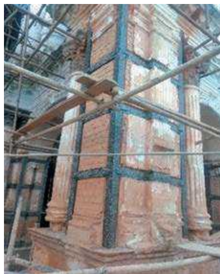
FIGURE 40: VERTICAL & HORIZONTAL METAL STRIPS IN BRICK PIER
