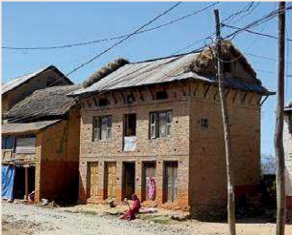
Photo 5: Brick masonry with cement mortar and CGI sheet roofing
