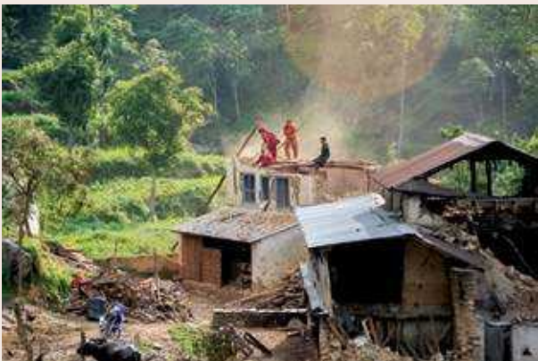
Photo 9: Owner-led demolition of house (Photo: Sandeep Gurung, 2015)
