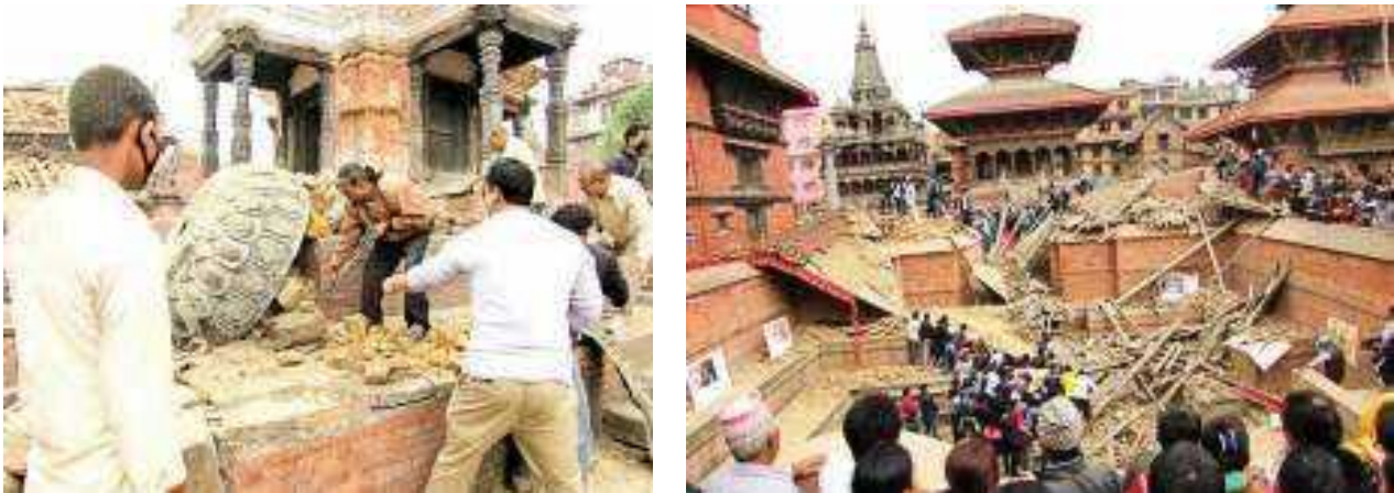
FIGURE 61: LEFT: PATAN DARBAR SQUARE. COMMUNITY ENGAGED IN RESCUING ARTEFACTS IMMEDIATELY AFTER THE EARTHQUAKE. RIGHT: RESCUE OF PEOPLE TRAPPED UNDER THE RUBBLE. PHOTOS: S. LAKHE. APR. 25, 2015.
