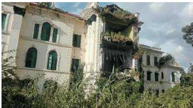
Collapse of south west corner
