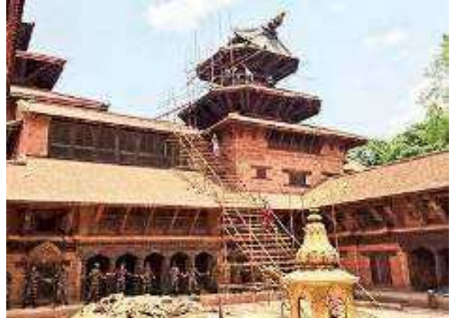
FIGURE 63: LEFT: VISVESHVARA TEMPLE, PATAN DURBAR SQUARE. TEMPORARY TIMBER SUPPORT WAS FIXED AT THE MONUMENTS THAT FACED STRUCTURAL RISKS. PHOTOGRAPH: R. RANJITKAR. MAY, 2015. RIGHT: NORTH TALEJU TEMPLE'S ROOF WAS DISLODGED. SCAFFOLDING WAS STARTED WITHIN A WEEK OF THE EARTHQUAKE AND THE TOP TIER WAS SECURED TO PREVENT FURTHER DAMAGE TO LOWER ROOFS. SOLDIERS ARE SEEN IN THE BOTTOM TRANSFERRING RESCUED BRICKS FROM THE SQUARE TO THE BACK GARDEN. PHOTO: R. RANJITKAR. MAY 10, 2015.
