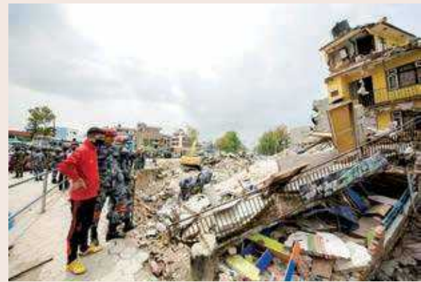
Photo 10: Armed Police Force and Nepal Army personnel working on demolition and debris management (Photo: Sandeep Gurung, 2015)
