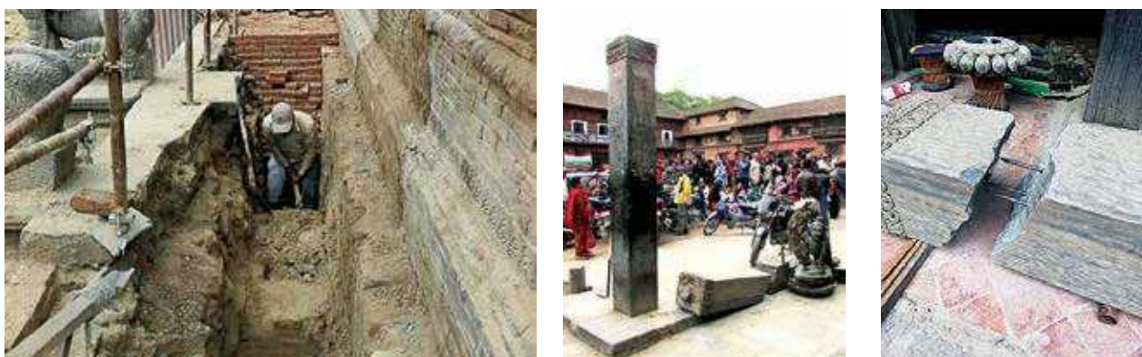
FIGURE 70: LEFT: NEW ADDITIONAL MASONRY WALLS IN MUD MORTAR USING MA-APA IN BETWEEN PLINTH WALLS, WHICH WAS FILLED WITH RUBBLE. PHOTO: KVPT. MIDDLE: BHIMSEN LION PILLAR HAD COLLAPSED IN THE EARTHQUAKE. PHOTO: S. LAKHE. APRIL 25, 2015. RIGHT: BROKEN PIECES WERE REPAIRED USING STAINLESS STEEL PINS TO JOIN BOTH ELEMENTS. PHOTO: KVPT. AUG. 2015.
