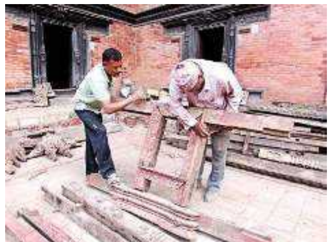
FIGURE 64: LEFT: THE SALVAGED WINDOW PARTS OF VARIOUS TEMPLES AND CARVED TIMBER ELEMENTS AND STRUTS WERE STORED IN A NEWLY BUILT SHED. PHOTOGRAPH: KVPT. JUNE 07, 2015. RIGHT: CARVED ELEMENTS WERE SORTED AND ASSEMBLED, AND ALL COMPLETE SETS FROM THE PILE OF RESCUED ELEMENTS WERE PLACED IN STORAGE. PHOTO: KVPT. MAY 02, 2015.
