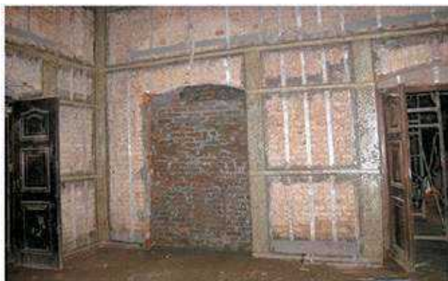
Carbon laminate and glass fibre used in retrofitting of wall
