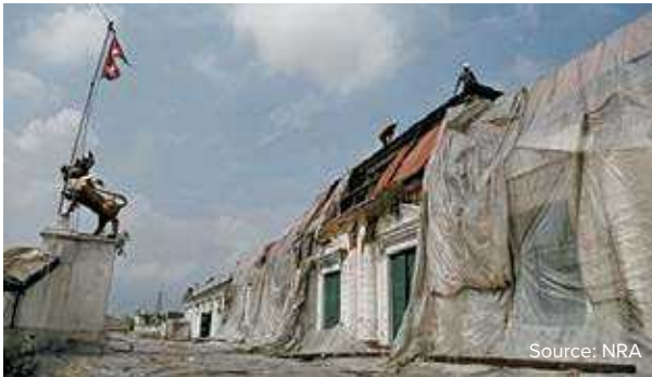
FIGURE 37: PROTECTIVE WORKS BEFORE RECOVERY
