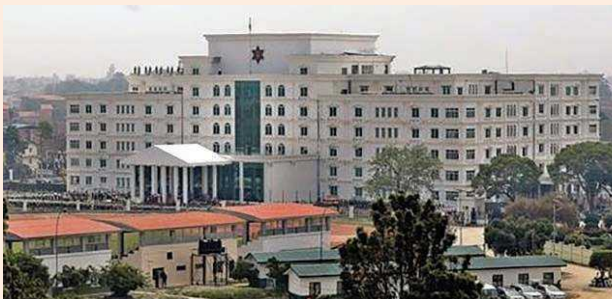
Photo 43: Army Headquarter after reconstruction
