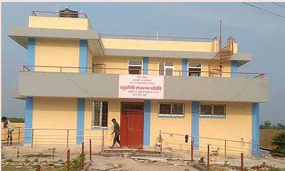
Photo 32: Completed health post building at Sukrauli, Nawalparasi
