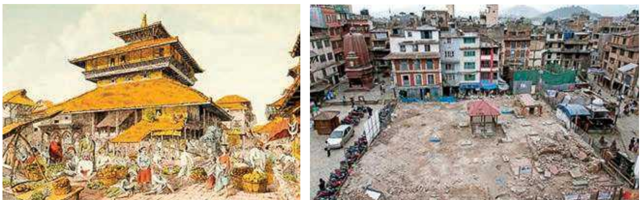
FIGURE 76: (LEFT) AN OLD PICTORIAL REPRESENTATION OF KASTHAMANDAP (CIRCA 1860S) AND (RIGHT) THE SITE OF KASTHAMANDAP AFTER REMOVAL OF DEBRIS.
