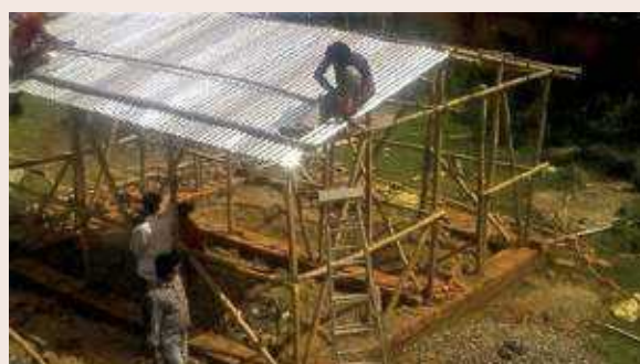
Photo 19: Model bamboo transitional shelter with necessary safety provisions (Source: NSET, 2015)
