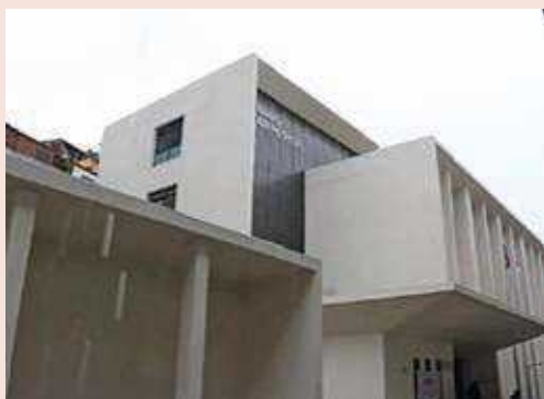
Photo 33: Bir Hospital, Kathmandu after reconstruction
